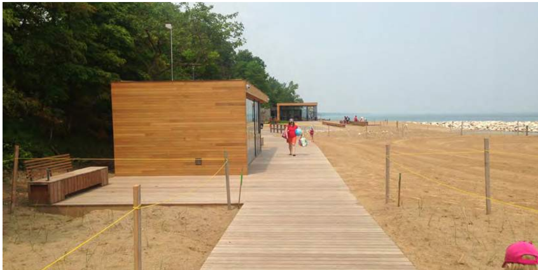
New boardwalk improvements.
