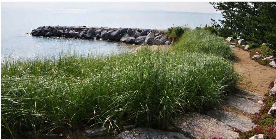
Example of stone breakwater structure and dune landscape.
