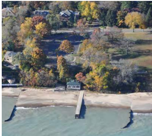
Stormwater management improvements.
