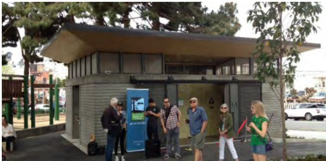
Example of a new upper level restroom facility.
