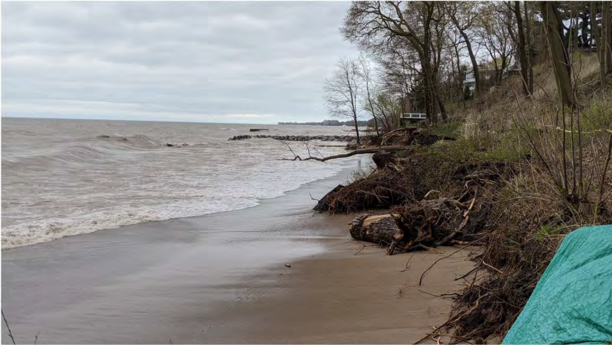
LLOYD PARK BEACH HOUSE LOOKING SOUTHEAST TO BLUFF 5/15/20
