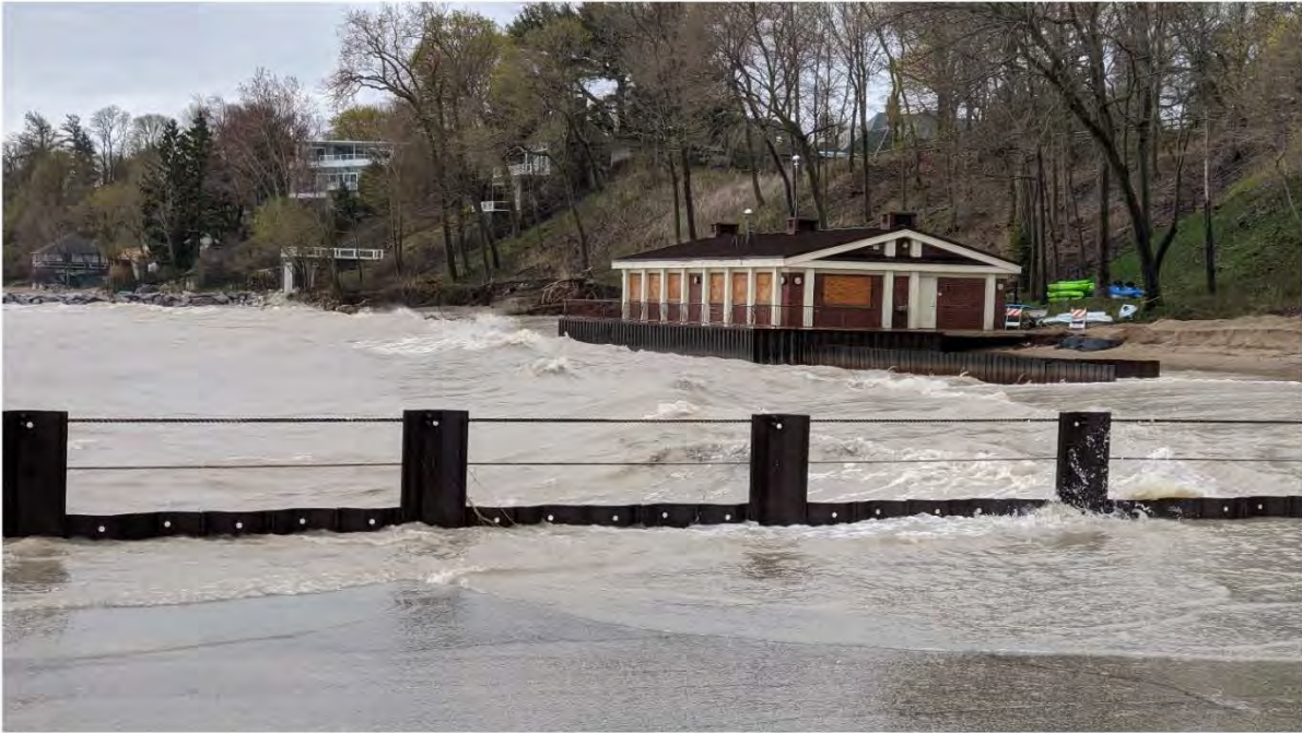
LLOYD PARK PIER LOOKING SOUTH TO BEACH HOUSE 5/15/2020
