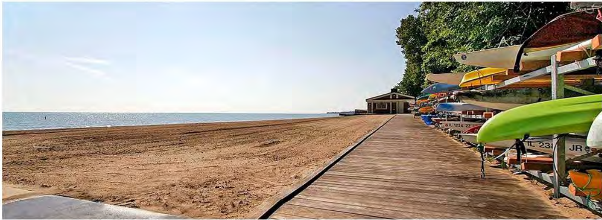
LLOYD PARK BOARDWALK & SAILBOAT RACKS LOOKING SOUTH TO BEACH HOUSE 5/2018
