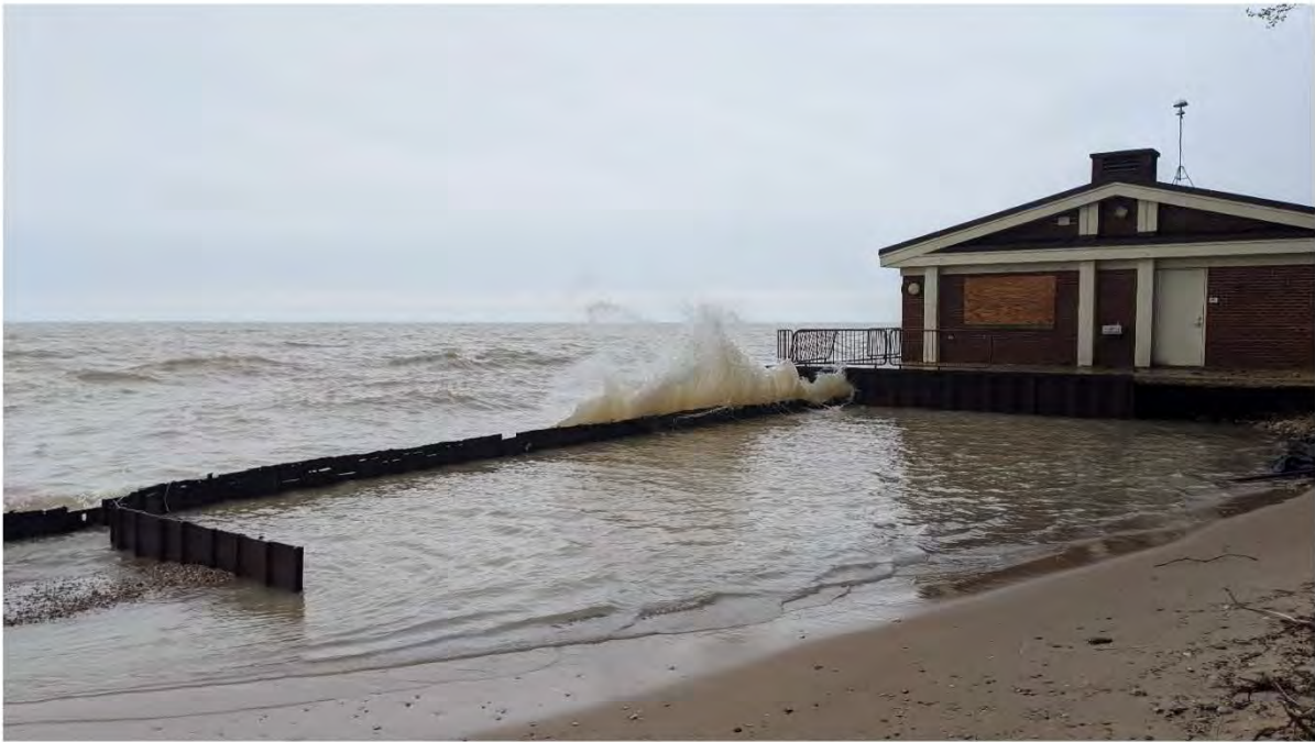
LLOYD PARK BOARDWALK LOOKING SOUTHEAST TO BEACH HOUSE 5/21/2020
