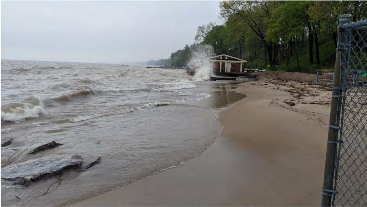
LLOYD PARK PIER LOOKING SOUTH TO BEACH HOUSE 5/21/2020
