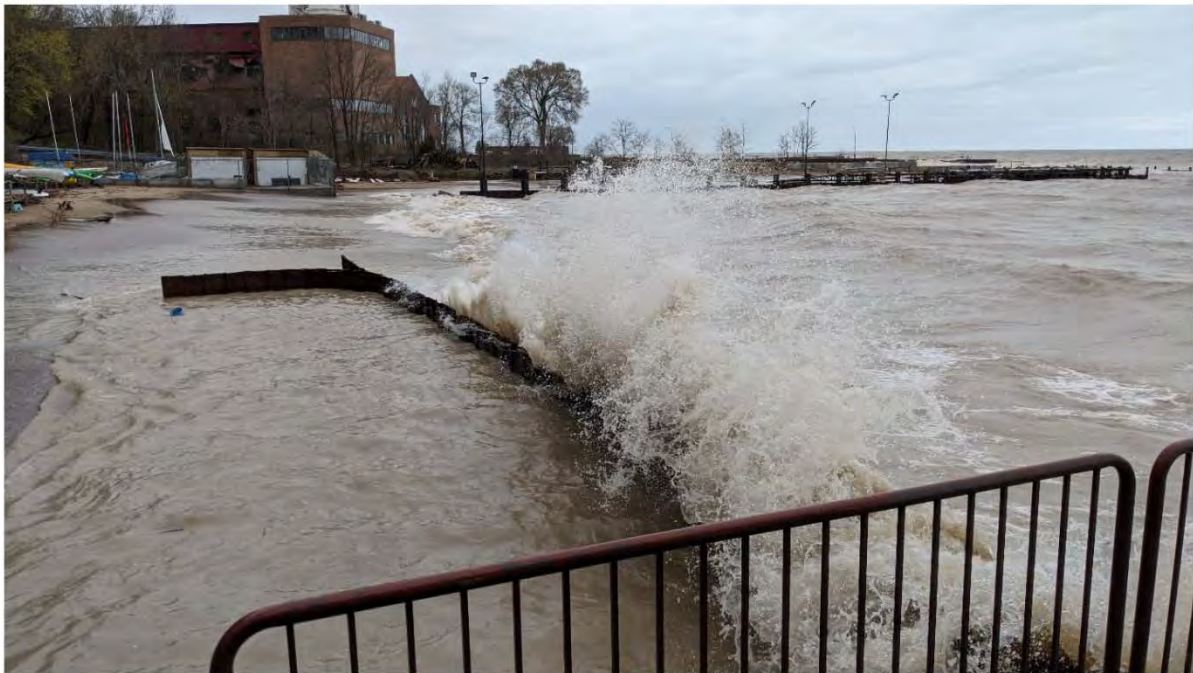
LLOYD PARK BEACH HOUSE LOOKING NORTH TO LAUNCHING PIER 5/15/2020
