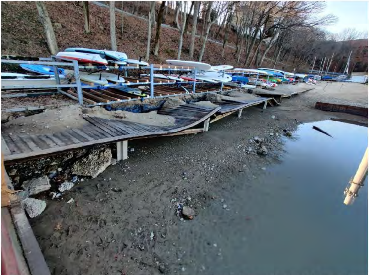
LLOYD PARK BEACH HOUSE LOOKING NORTH TO BOARDWALK & SAILBOAT RACKS 12/2019
