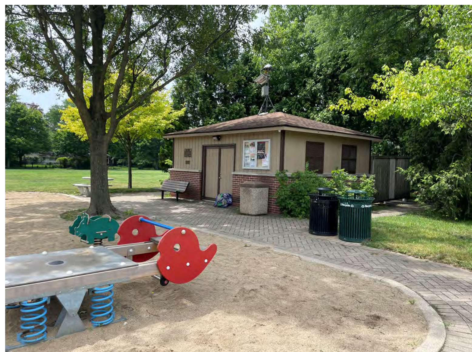
EXISTING BUILDING LOOKING SOUTHWEST
