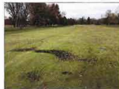
BEFORE: LACK OF EXISTING FAIRWAY SLOPE DOES NOT ALLOW SURFACE DRAINAGE FLOW TO EXISTING DRAINAGE INLETS.
