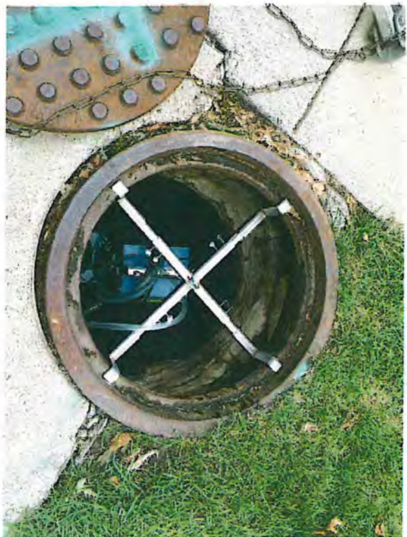
Installation within manhole using hanger.
