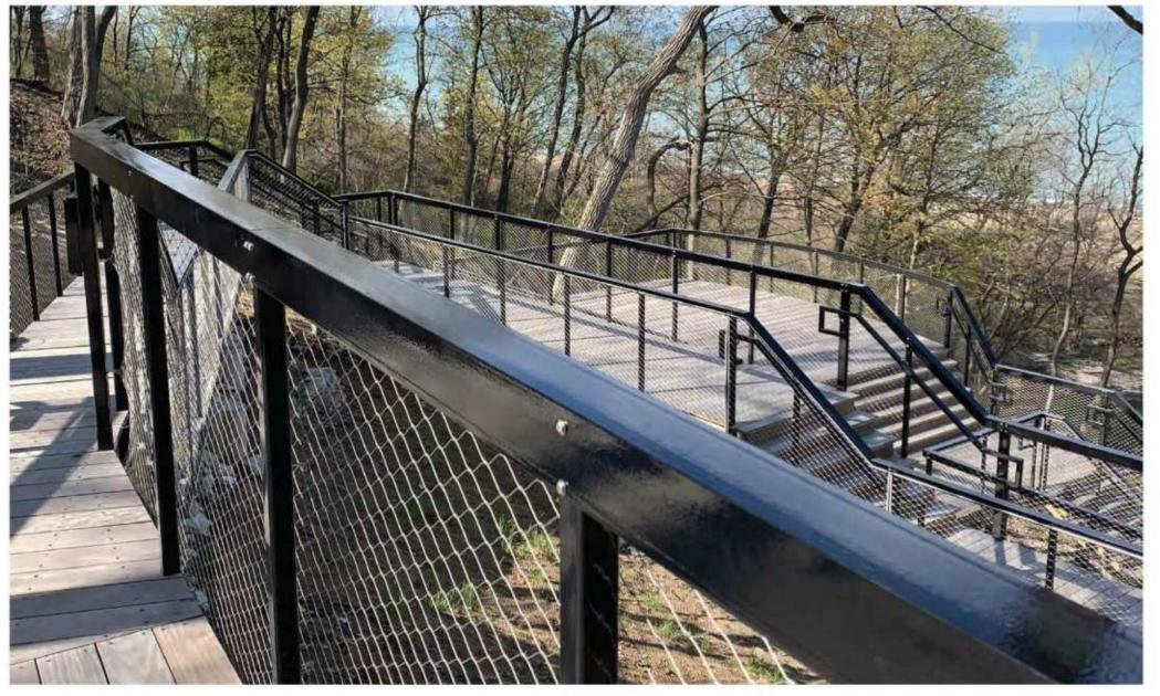
**GUARDRAILS & FENCING** METAL POST, XTEND MESH
