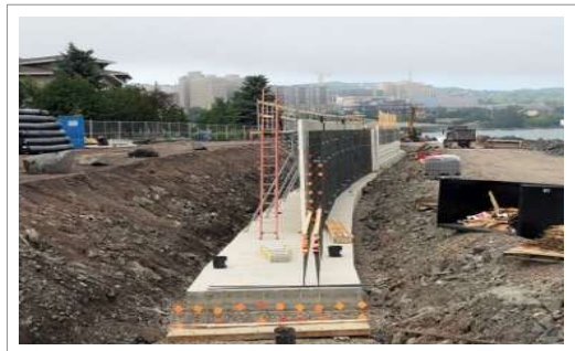
Concrete Walls Construction
