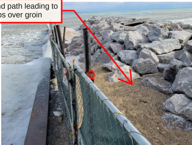
Accreted sand between steel & stone groin, Feb-9-2025
