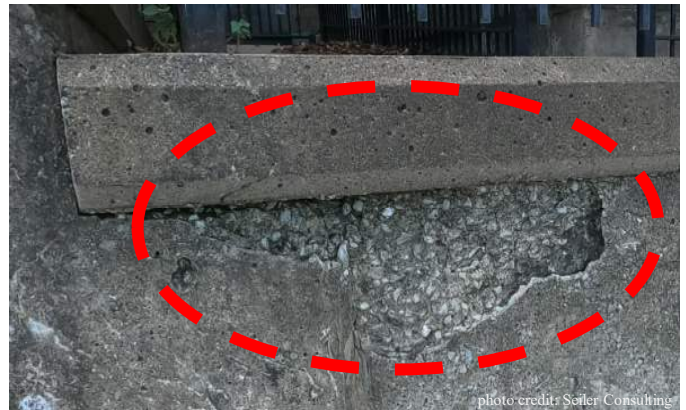
Spalling concrete sea wall
