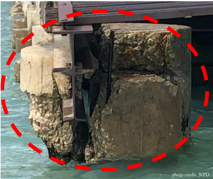
Damaged pier
