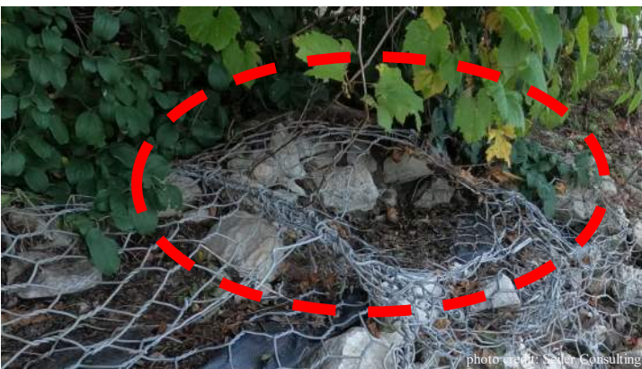
Damaged gabion basket
