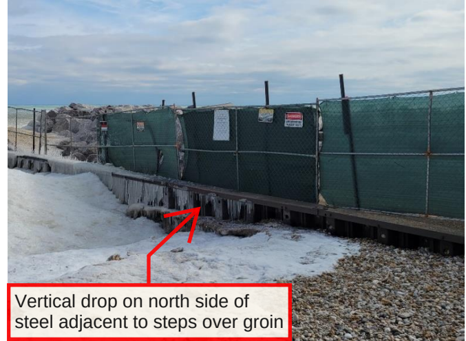
Sand level at Centennial South Groin, Feb-9- 2025
