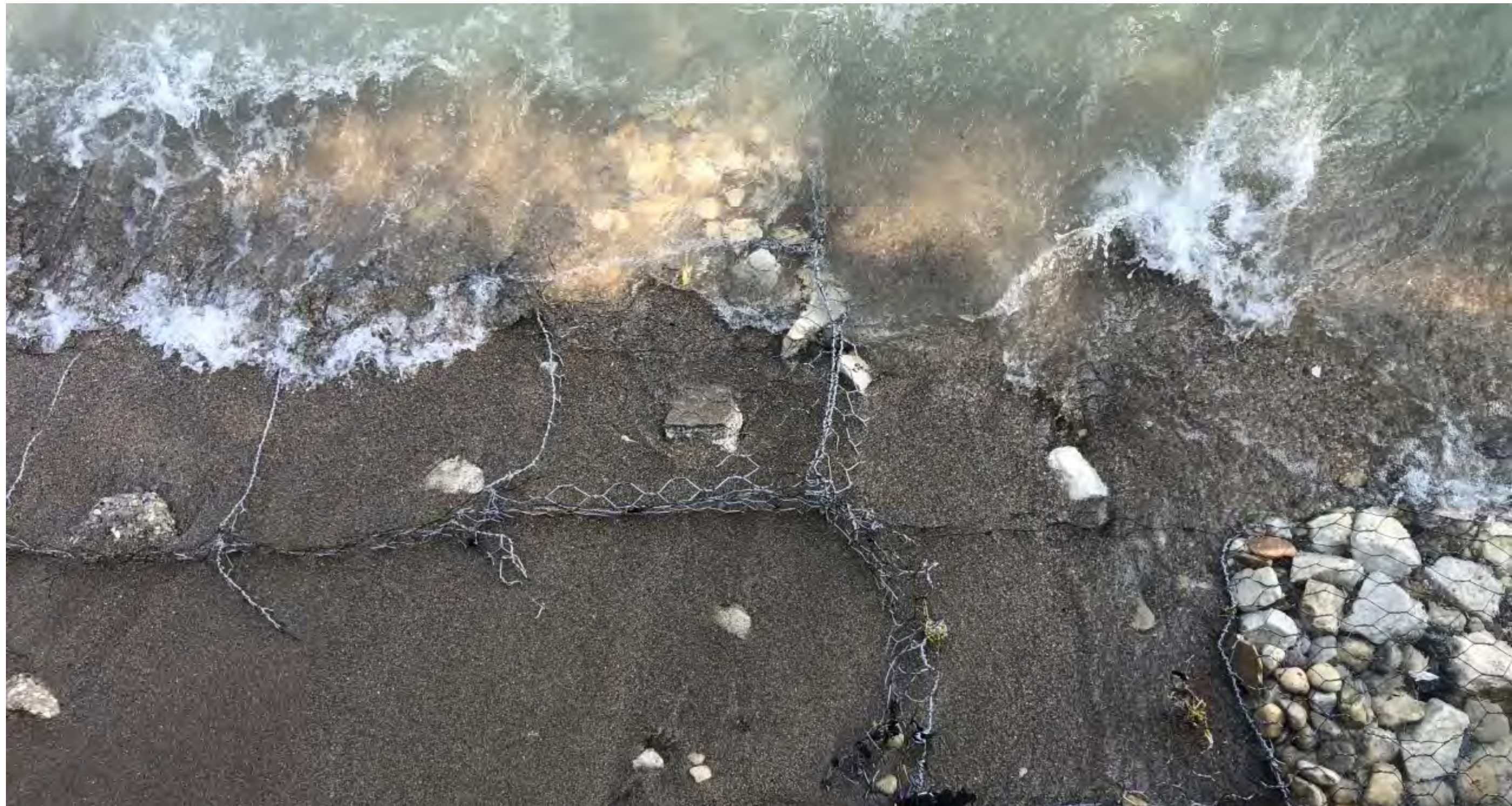
ELDER LANE | FAILING GABION BLANKETS OCTOBER 2020
