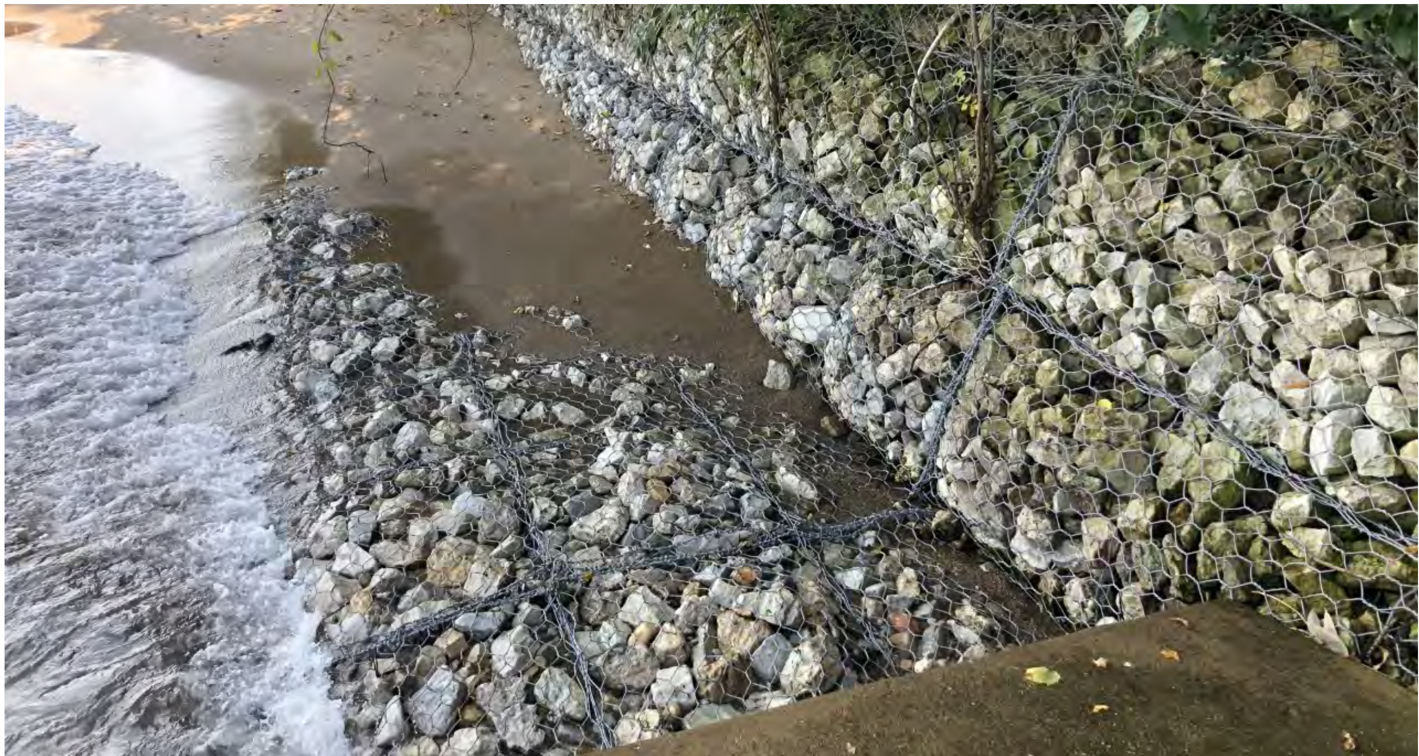
ELDER LANE | FAILING GABION BLANKETS OCTOBER 2020
