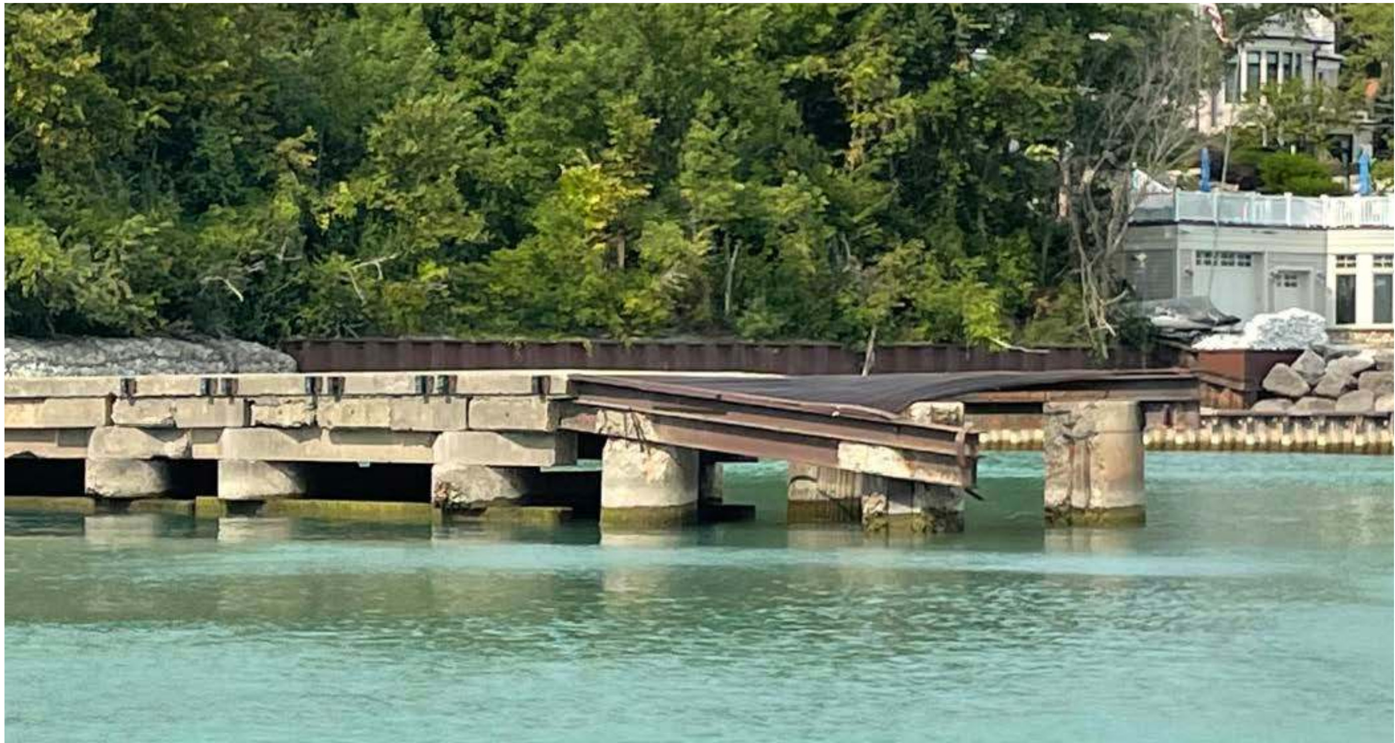
ELDER LANE | FAILING PIER SEPTEMBER 2020
