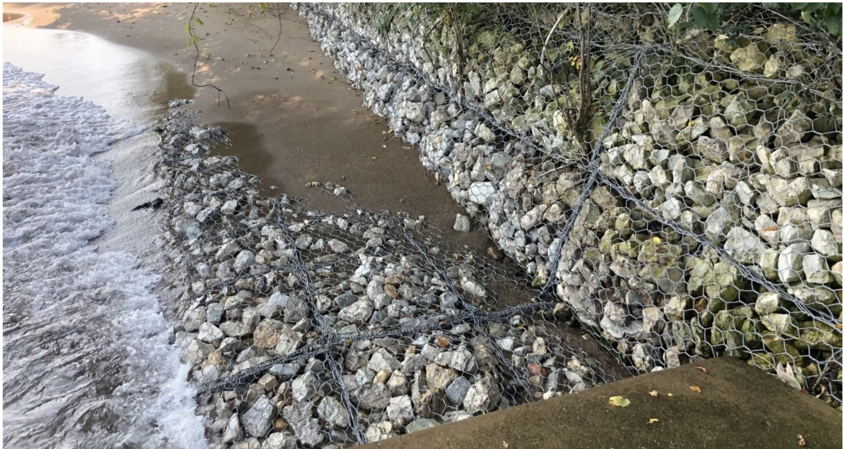
ELDER LANE | FAILING GABION BLANKETS OCTOBER 2020
