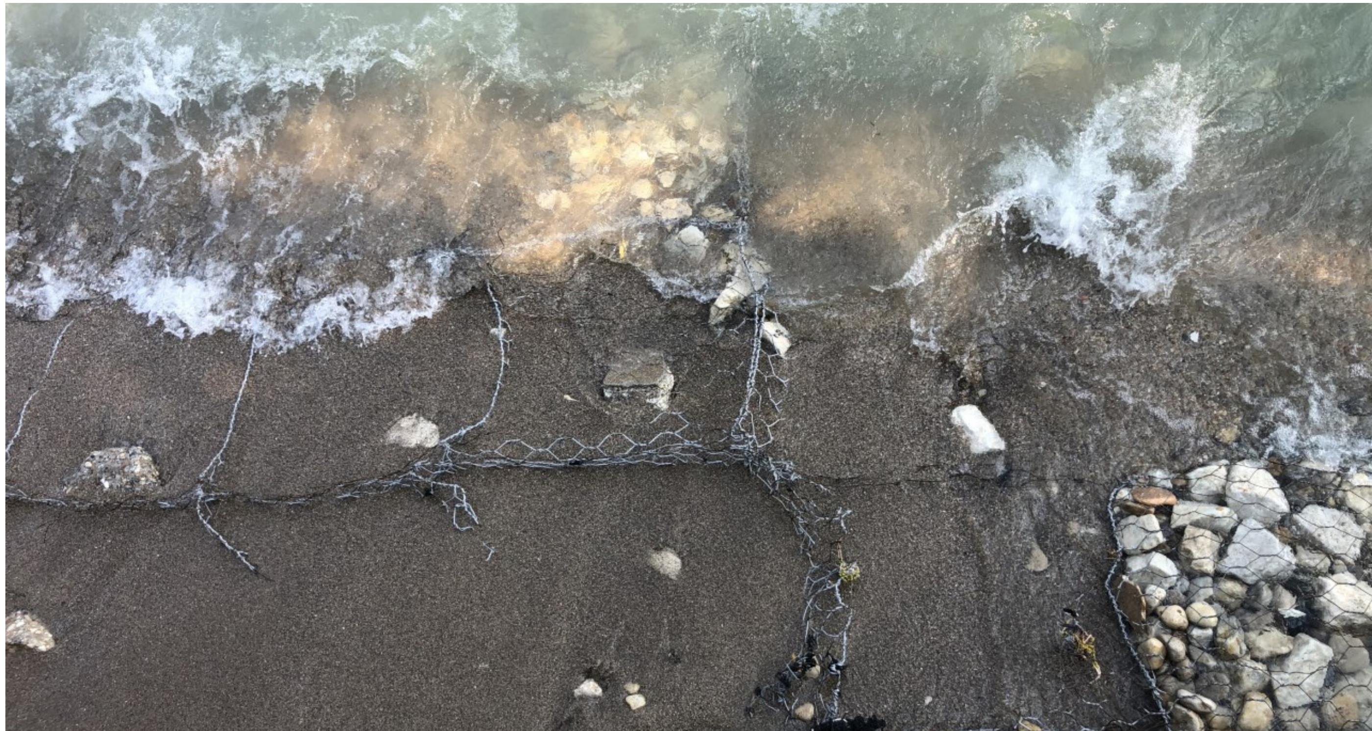
ELDER LANE | FAILING GABION BLANKETS OCTOBER 2020
