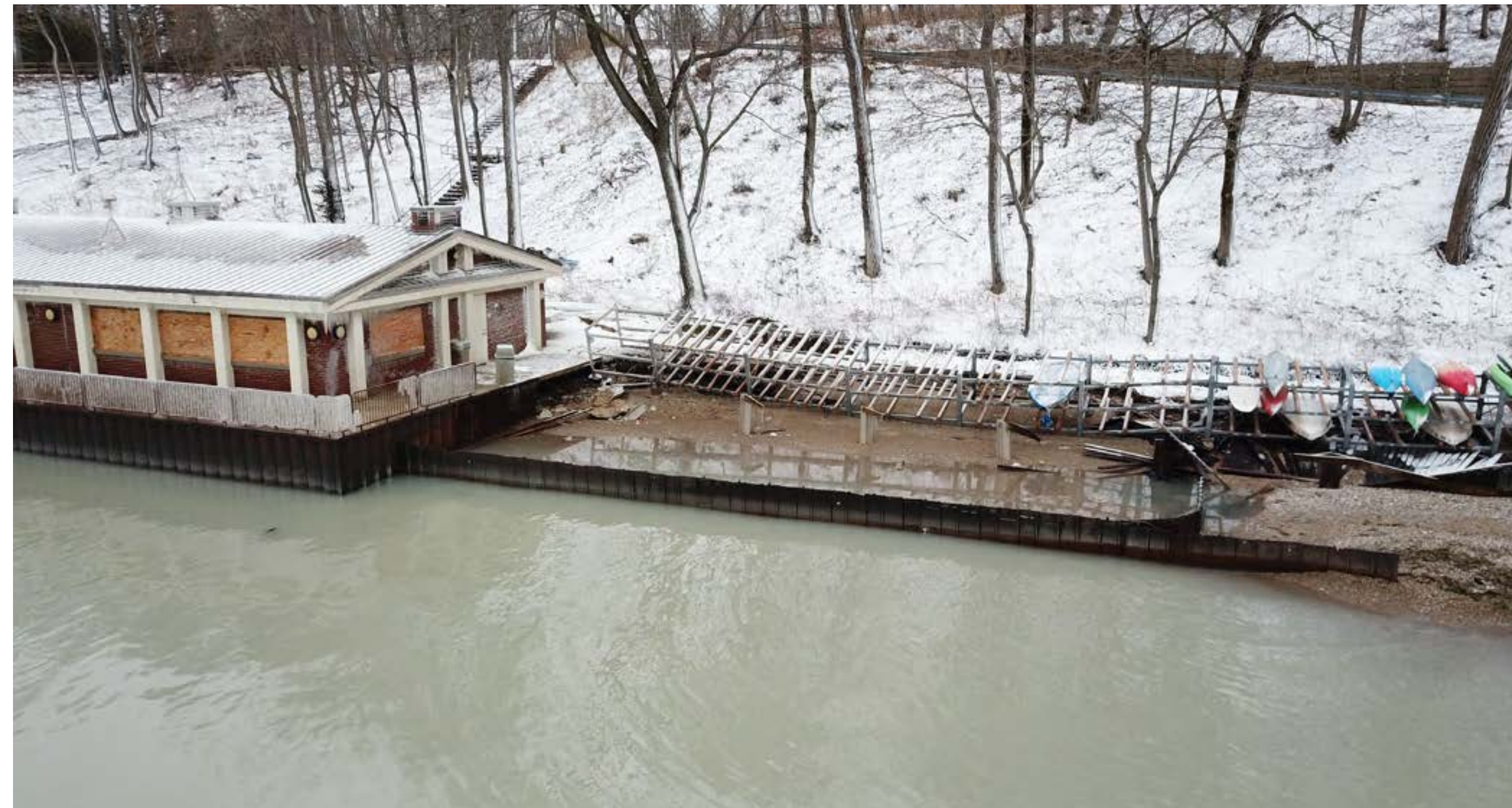
LLOYD STEEL SHEET PILE IN FRONT OF BOAT RACKS | ELEVATION 584.4 OCTOBER 2019
