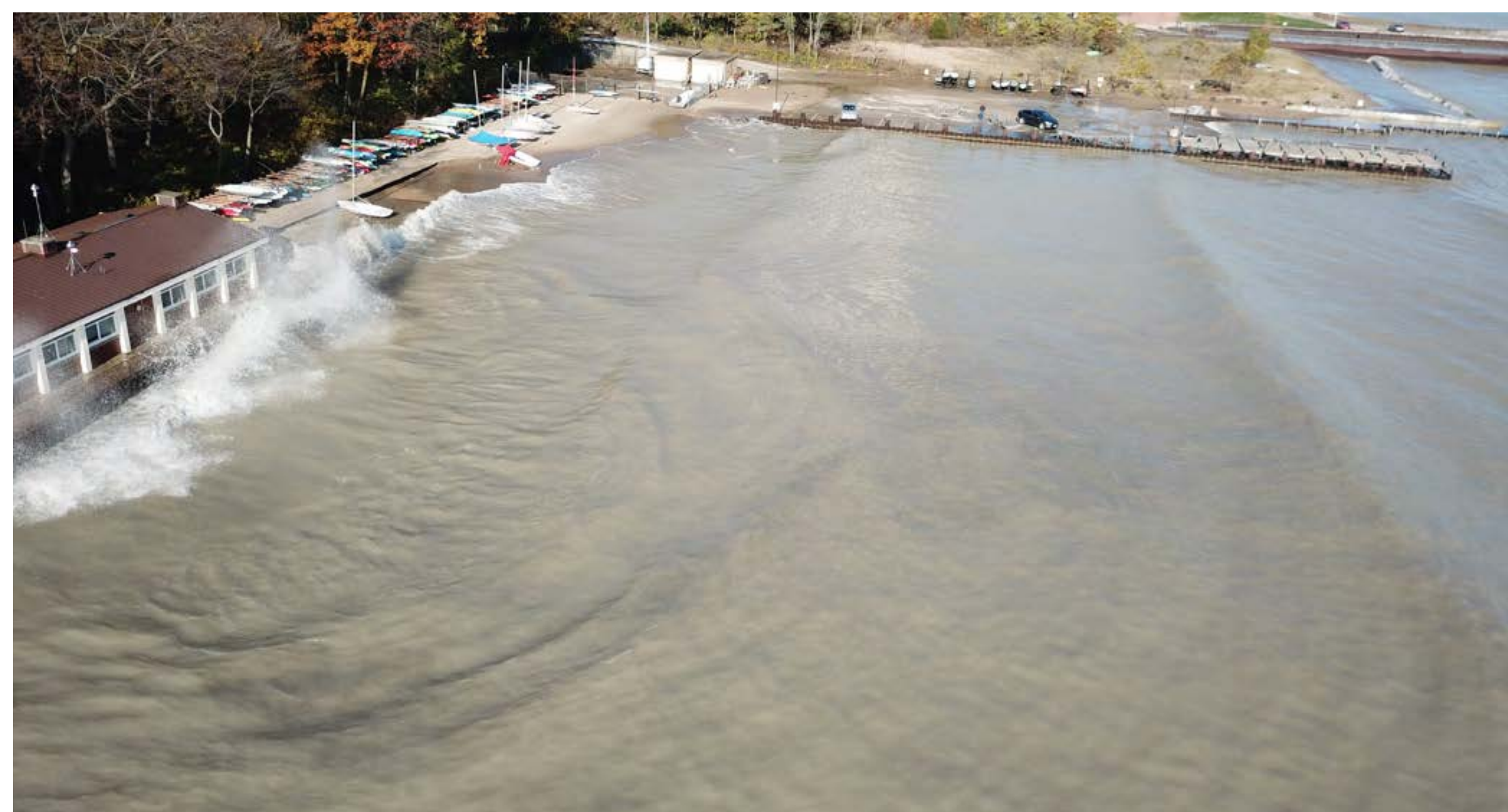
LLOYD BOAT HOUSE SHEET PILE + CONCRETE WALL | ELEVATION 586.5 OCTOBER 2019
