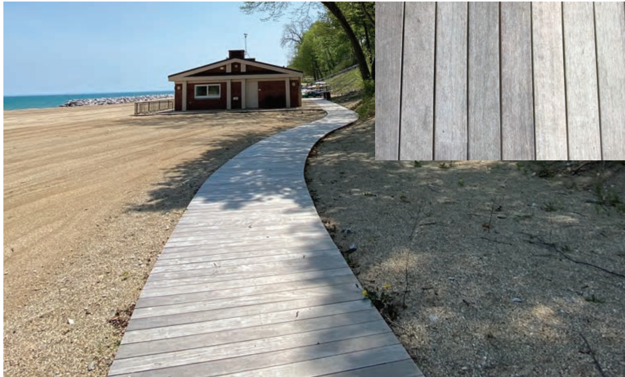
IPE BOARDWALK DURABLE NATURAL DECKING, FADES TO SILVER GRAY MATERIAL VERNACULAR USED THROUGHOUT WINNETKABEACHES
