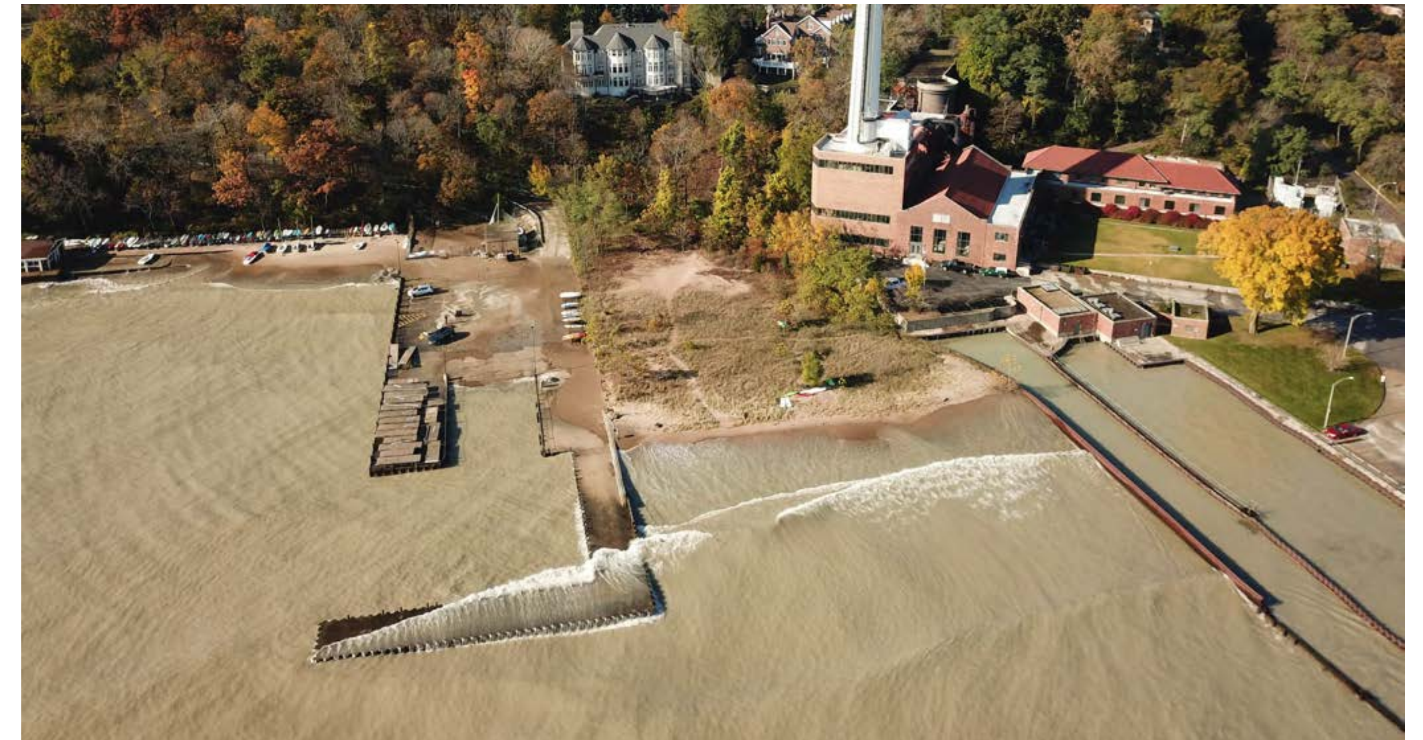
LLOYD PIER | ELEVATION 583.3 OCTOBER 2019
