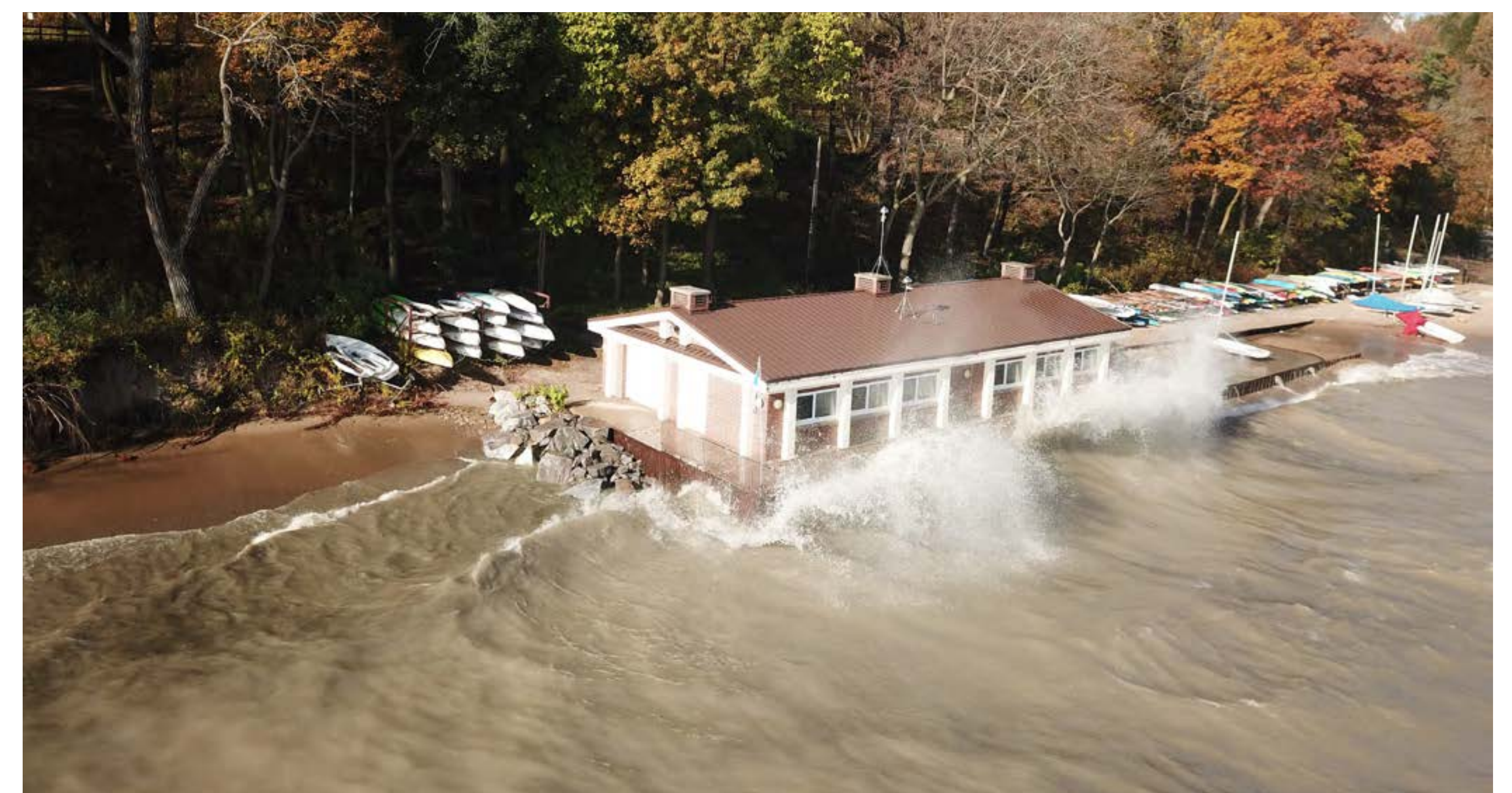
LLOYD BOAT HOUSE SHEET PILE + CONCRETE WALL | ELEVATION 586.5 OCTOBER 2019
