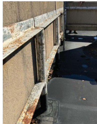
E-6: Administration Building: steel structure at screen panels rusting
