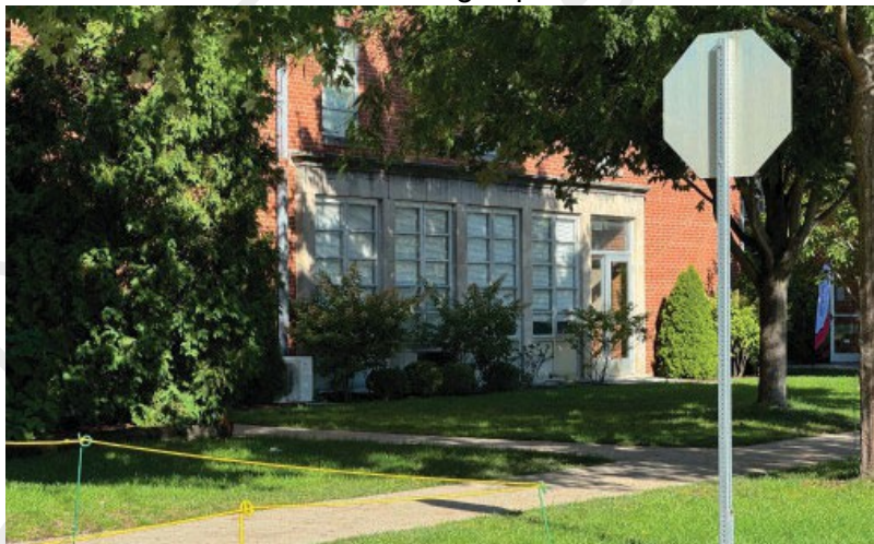
A-2A: A. C. Nielsen Tennis Center: windows and storefront needing replacement
