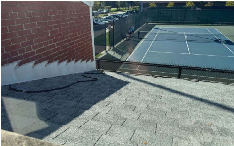
A-3A: A. C. Nielsen Tennis Center: heat trace cables
