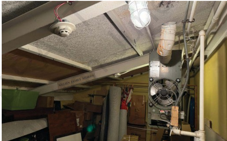
A-3B: A. C. Nielsen Tennis Center: uninsulated underside of roof
