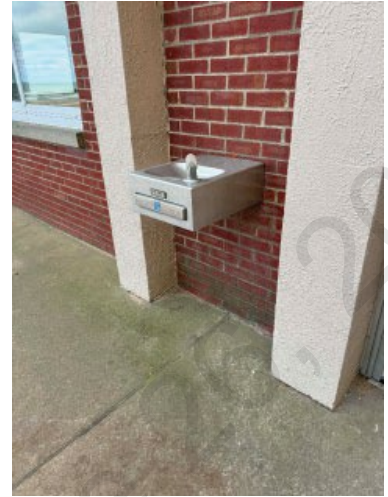
J-2and3: Lloyd Beach House: non-ADA compliant water fountain with mildew below
