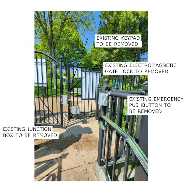
**EXISTING GATE ACCESS EQUIPMENT TO BE REMOVED** N.T.S.
