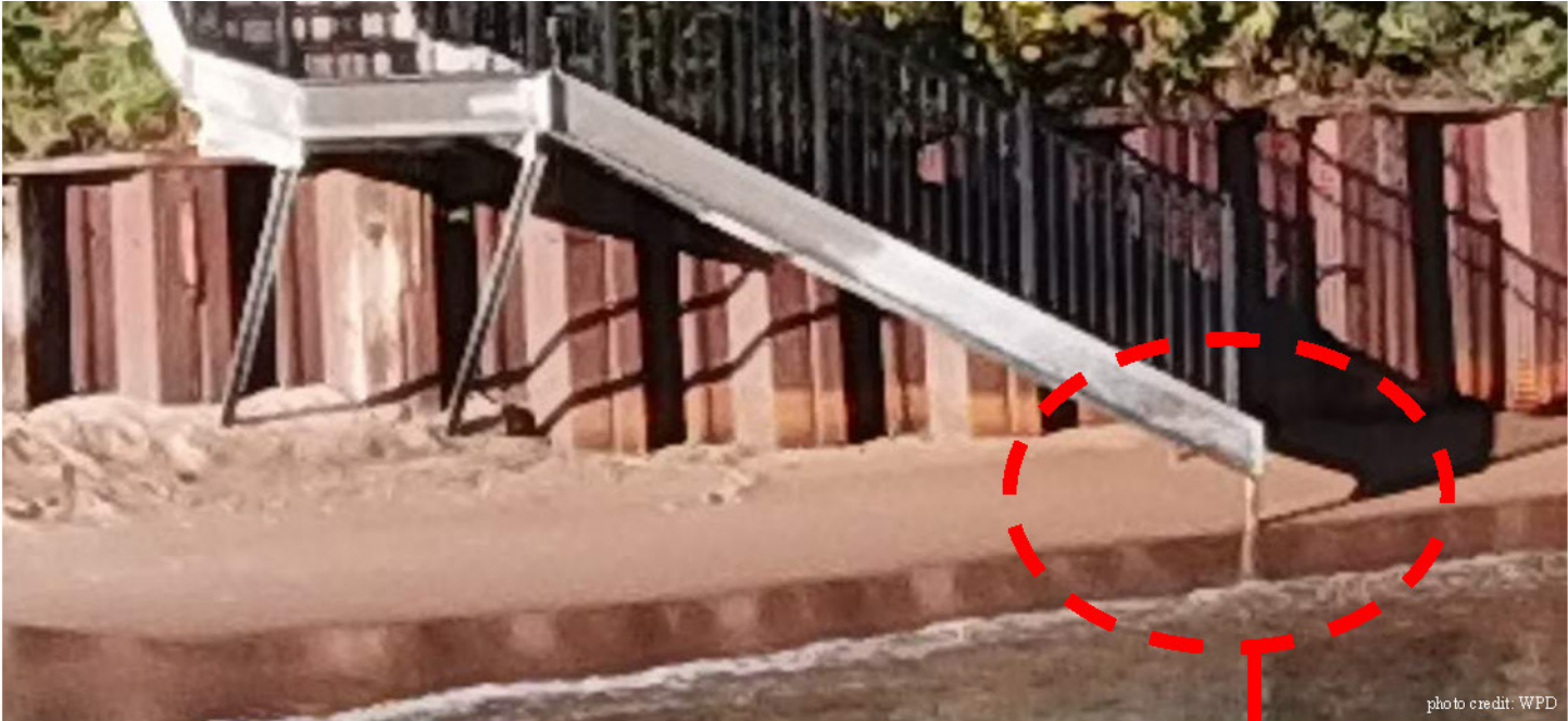
Beach erosion in 2020 meant stairs ended 24" above the beach level
