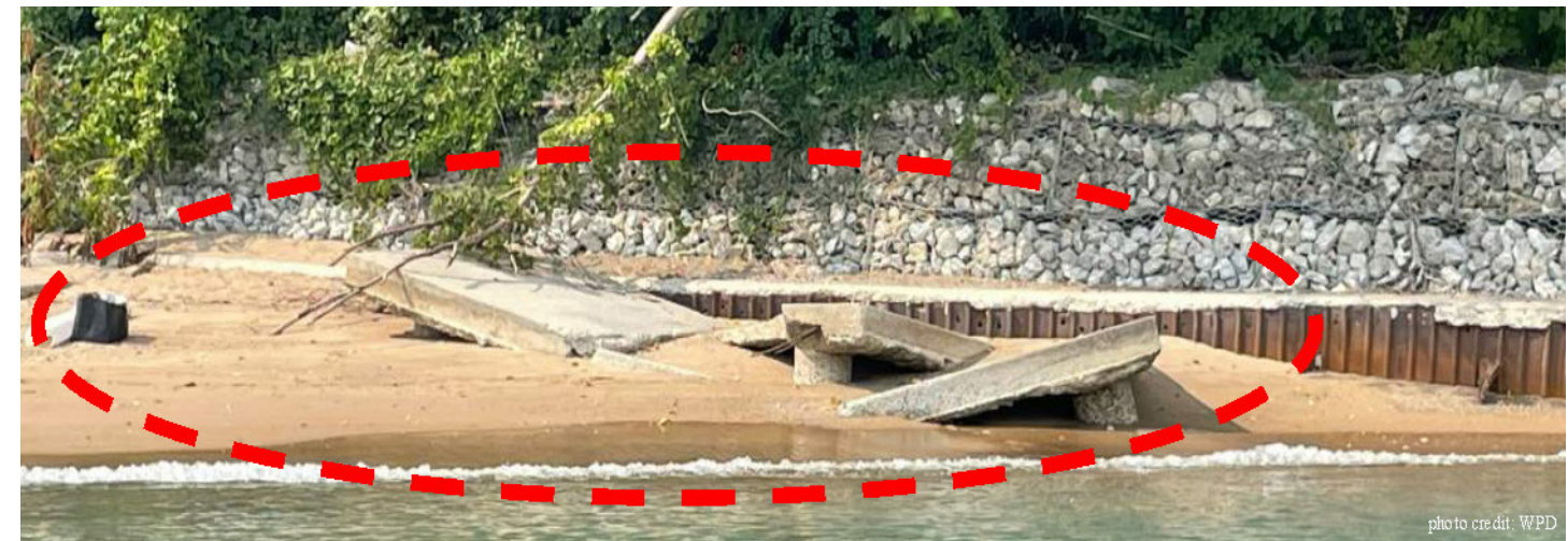
Damaged kayak storage rack foundations
