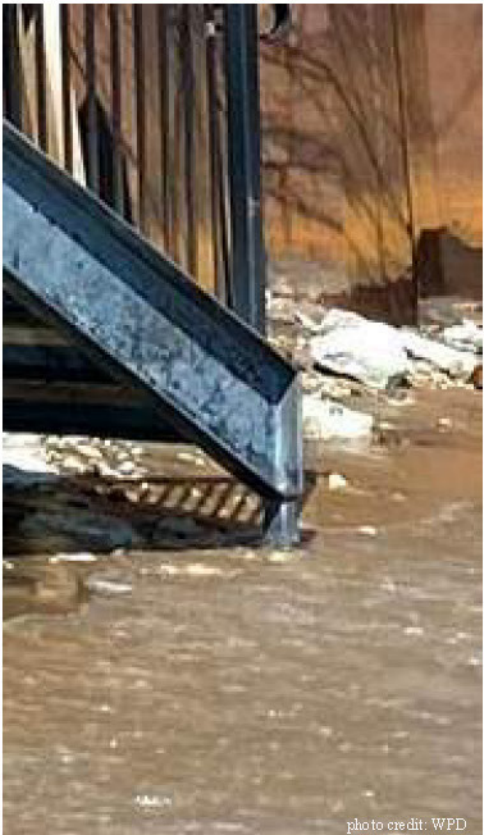
Beach erosion in 2020 meant stairs ended 24" above the beach level
