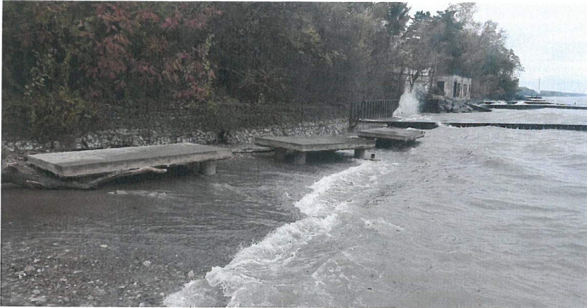
2020 photo looking north at the damaged non-motorized storage pads and gabion baskets, existing steel groin and north shoreline structures
